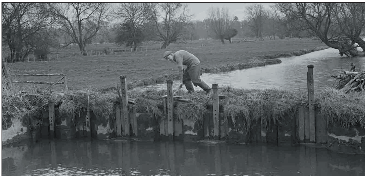
A 'drowner' at work on a seven-hatch weir at Lower Farm, Britford, 1954.
