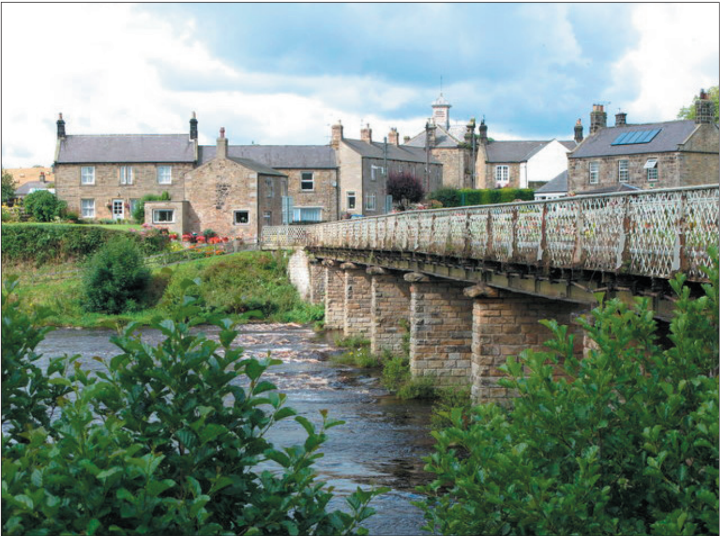
Wark Bridge, opened 27 August 1858.
