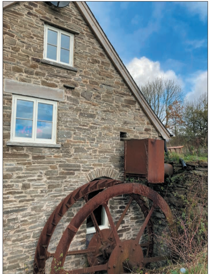
Outside Rhosgoch Mill showing the wheel.
